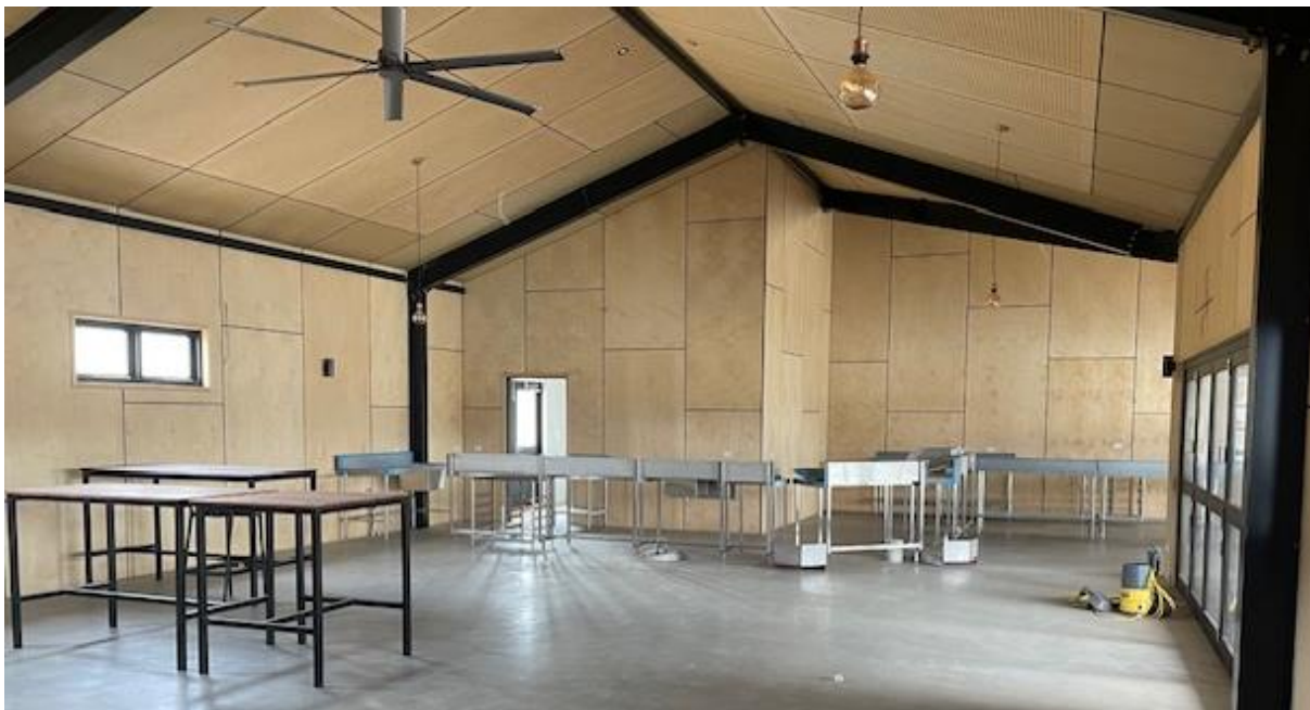
Bar area with bar module in position
