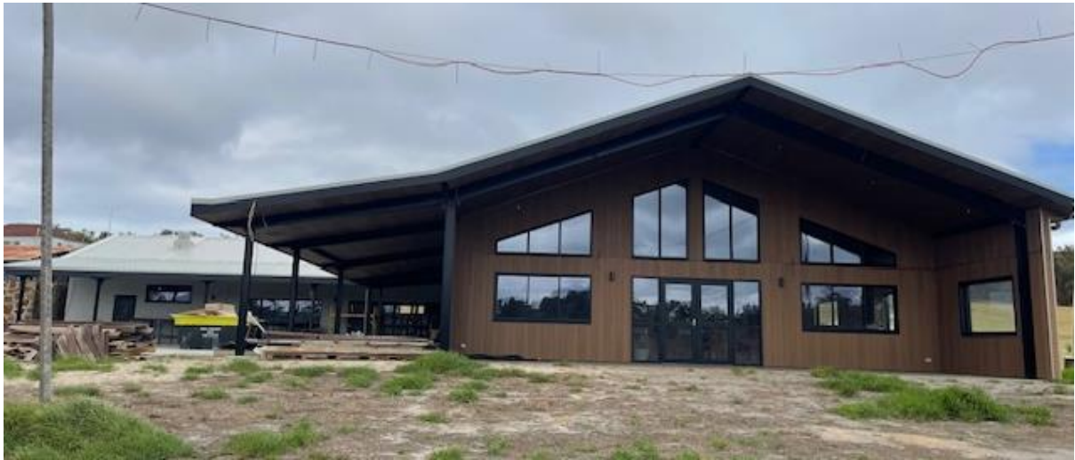
Work in Progress of New Building
